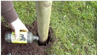
Kongcrete® is a hydrophobic (insensitive to water) two-part composite backfill that expands to fill the peripheral void between a fence or sign post and the hole. Kongcrete® expands immediately after mixing and reaches 50% of full strength in approximately 3 minutes. The product completely sets in approximately 2 hours.
